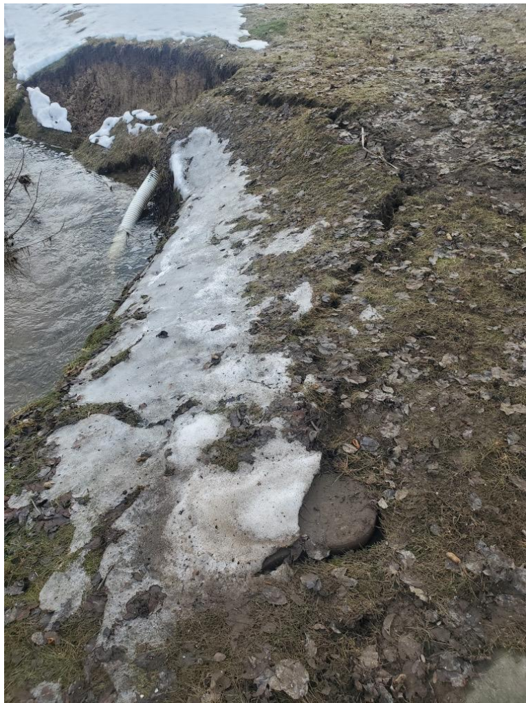
current bank erosion
