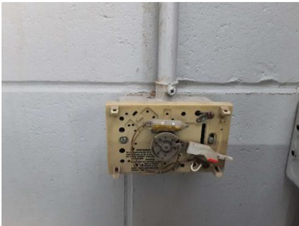
Liquid mercury ampules present within thermostat
