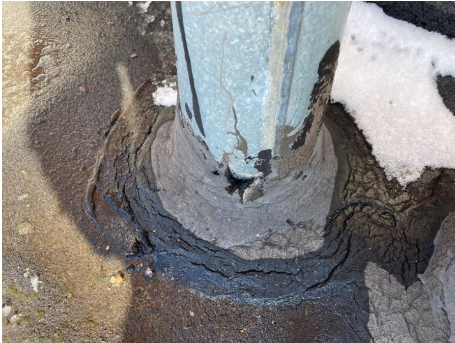
Photo 1 - Non-asbestos black tar and grey caulking at roof penetrations
