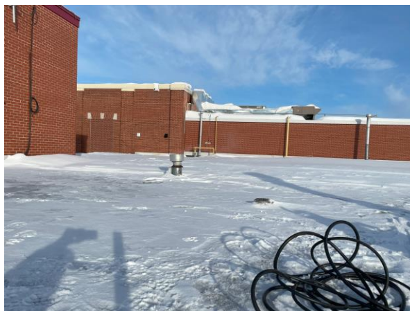
Non-asbestos built up roofing, Main Roof
