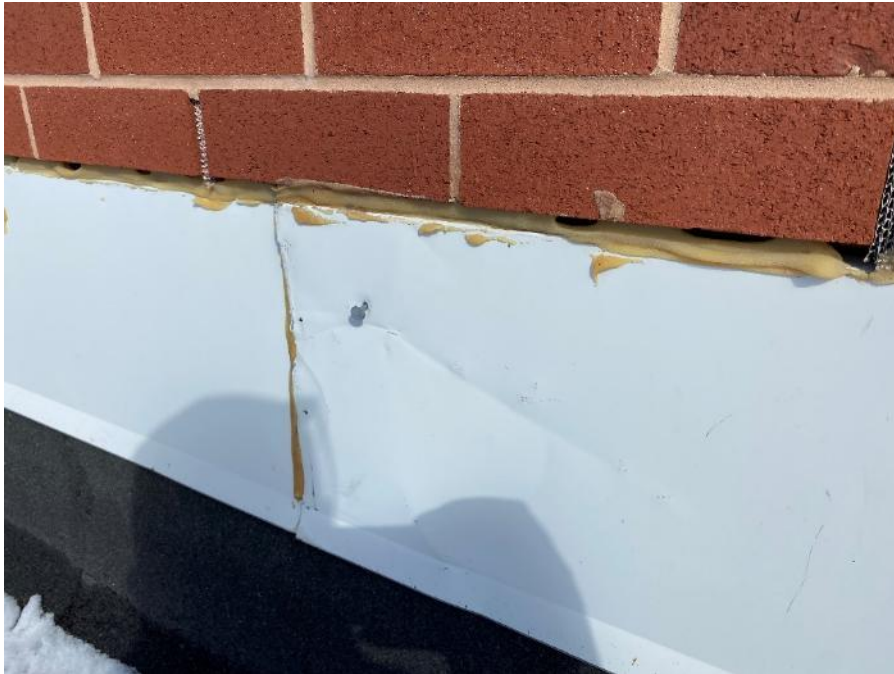
Photo 3 - Non-asbestos yellow caulking on flashing
