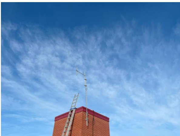
Non-asbestos built up roofing, Upper Roof
