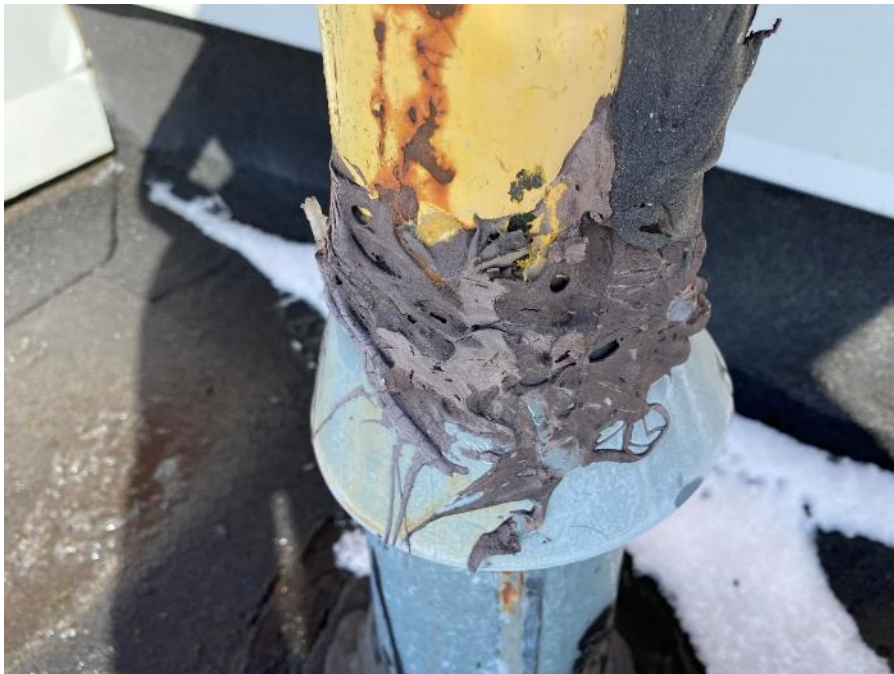
Photo 2 - Non-asbestos grey caulking at pipe penetrations
